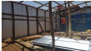
..... the latest classroom extension
