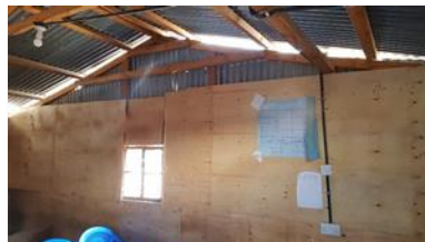
... with Safe sockets and new electrics
